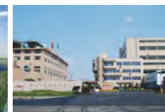
TBR Plant in Xiasha
